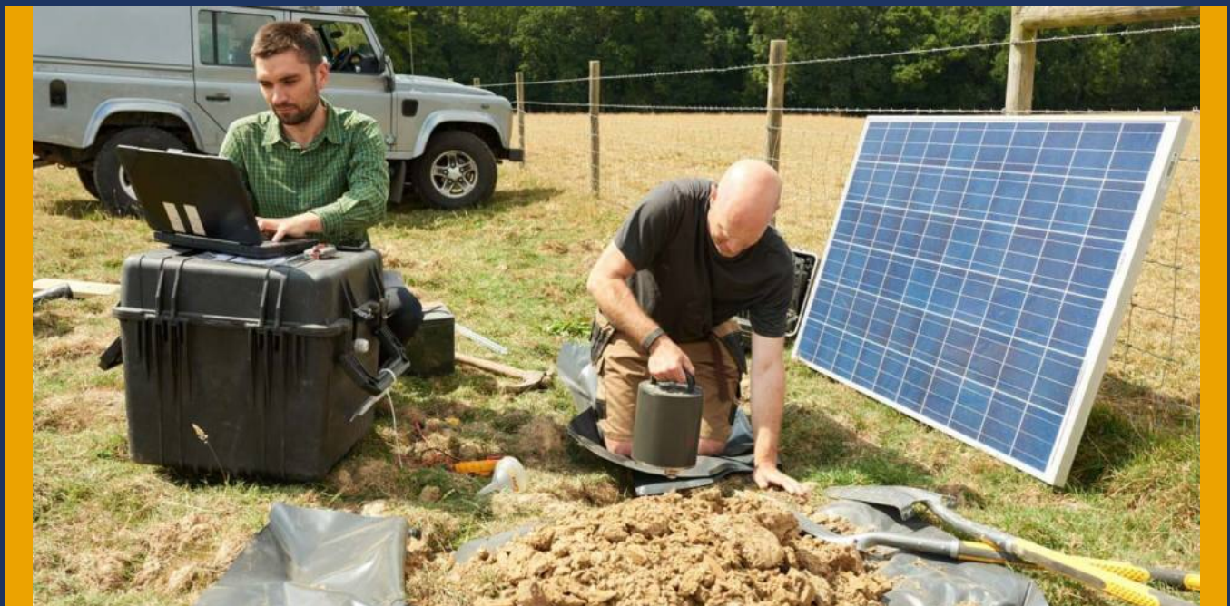
Seismometer installation in the field to monitor for earthquakes. This is an important part of establishing natural baseline conditions and can identify impacts of human activity in the subsurface. Credit: BGS © UKRI
